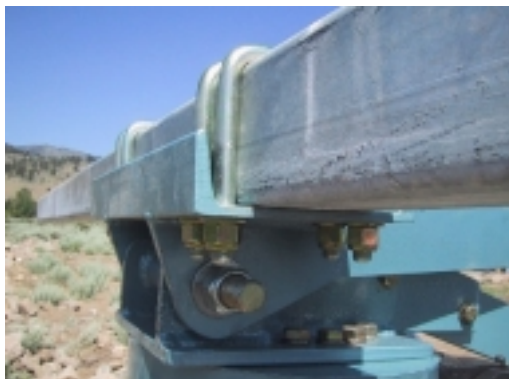
TIGHTEN NYLOCK 5/16" U-BOLT NUTS EVENLY .
