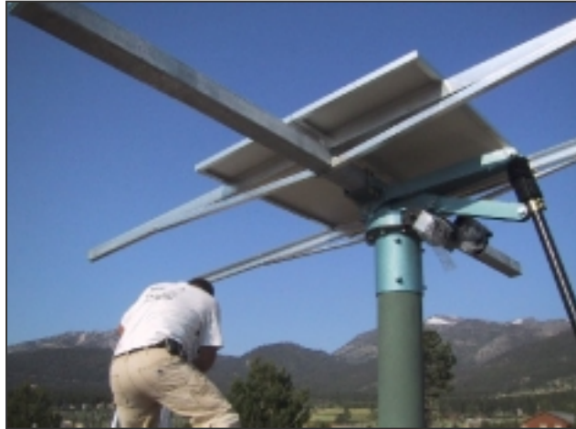
One installer, one piece at a time approach. Modules are being used to “square-up: the frame. Notice how the modules overhang the Rails.
