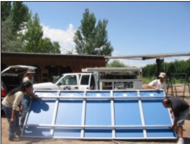
Sub-Array Approach: Requires a lot of people power. Notice that the rails bolt to the intermediate module holes. Lift by the tracker rails only, not the module frames!
