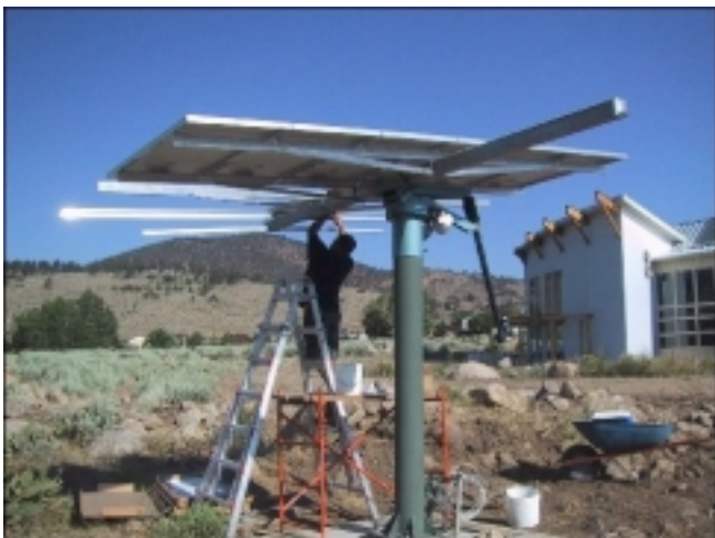
Sub-Array Approach: Requires a lot of people power. Notice that the rails bolt to the intermediate module holes. Lift by the tracker rails only, not the module frames!
